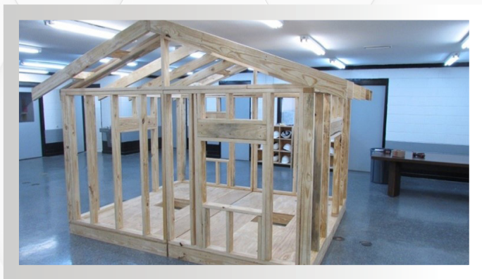
Small scale test built by the carpentry students
